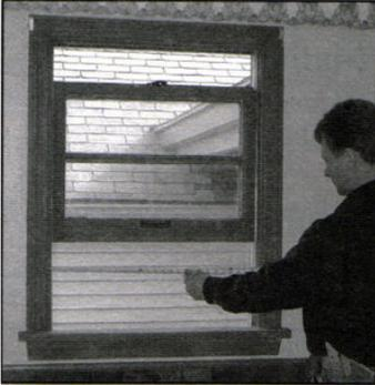
The new window is anchored to the old window frame against the exterior or blind stop, larger interior stops (must be purchased) are reinstalled to complete the installation.
