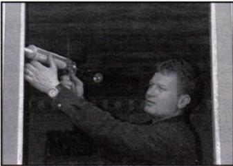
3. Caulk the inside edge of the blind stop along the top and down both sides. Make the caulk bead about 1/8". The bead should not lie against the window frame, just the blind stop. Place a bead of caulk on the top of the expander.
